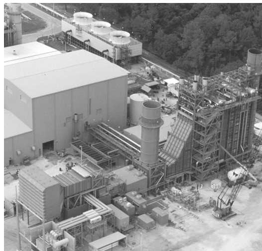
Cane Island Unit 3 is a 250 MW combined cycle generating unit, which began commercial operation Jan. 25. The unit is owned equally by FMPA and the Kissimmee Utility Authority.
